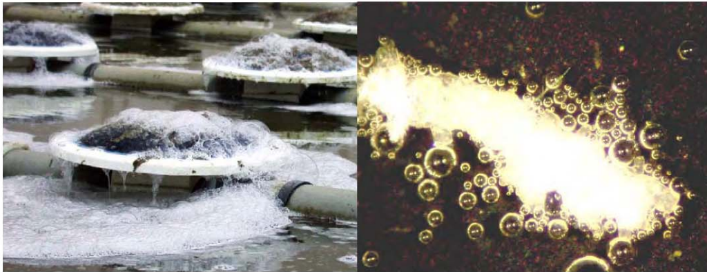
Figure 9: Cleaning of EPDM-membranes
